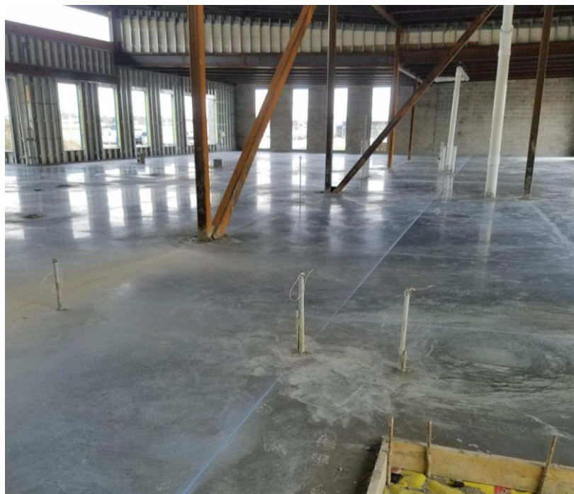
Project Site on November 3, 2018
