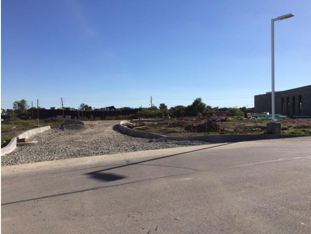
Project Site on October 17, 2018 View of the entrance drive with new curbs. Approximately 80% of the site concrete has been installed.
