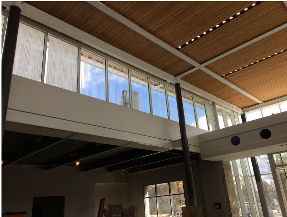
Project Site on November 6, 2018 View of the Concourse with the installation of the window film.
