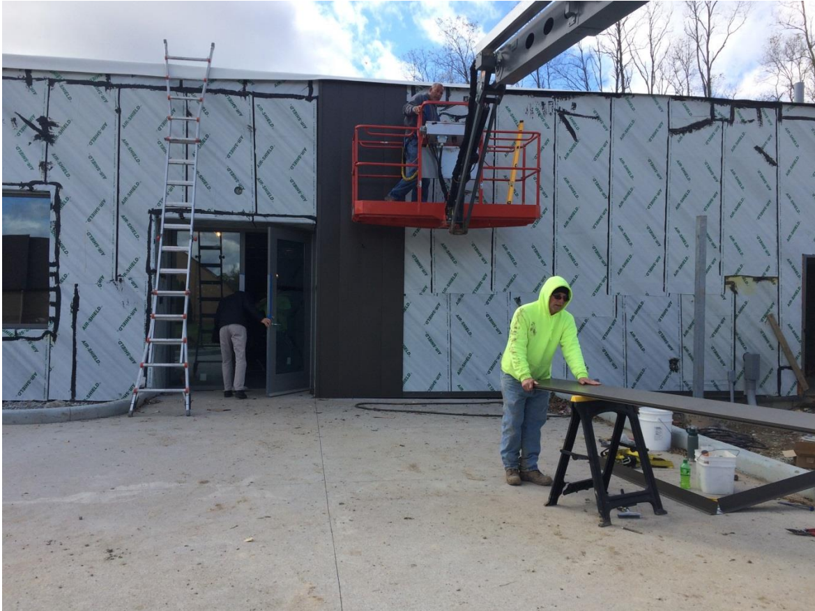
Project Site on November 6, 2018 Installation of the metal panels on the east elevation.
