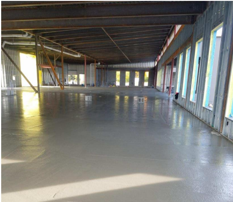
Project Site on November 3, 2018
