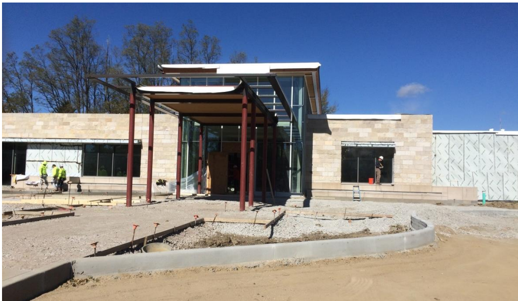
Project Site on October 23, 2018 View of the entrance with curbs and planters installed.
