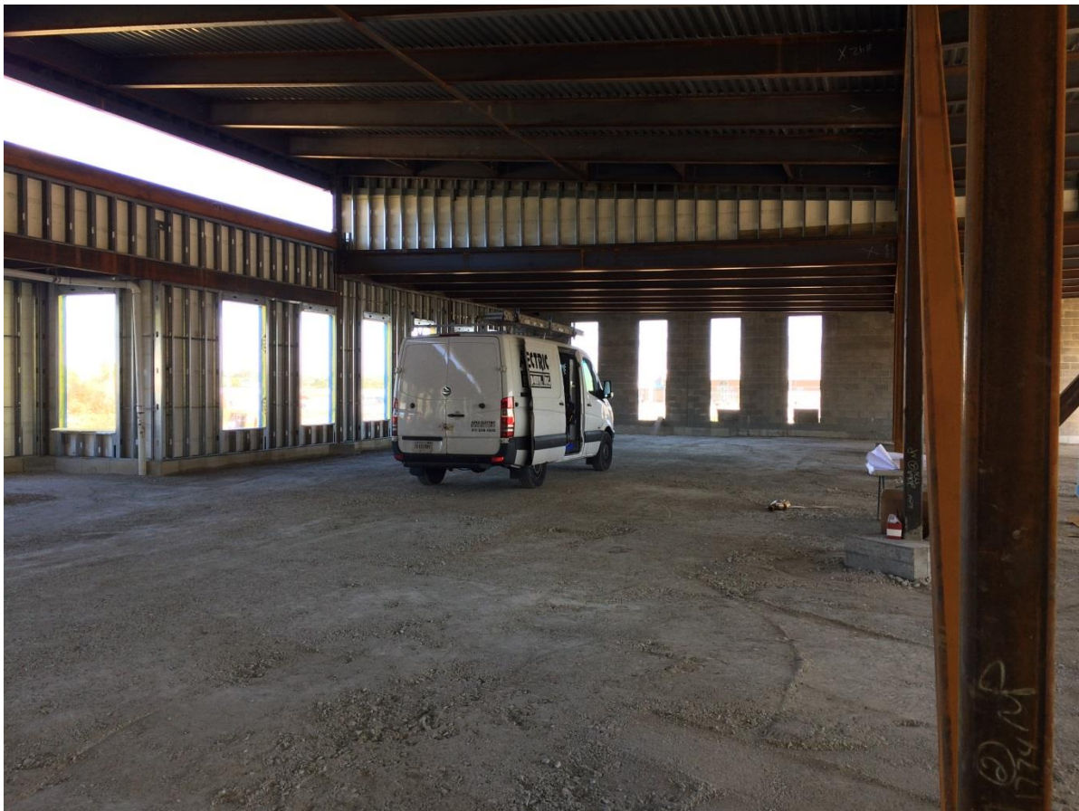
Project Site on October 31, 2018 View looking east with concrete slab stone base and electrical rough-ins in process.
