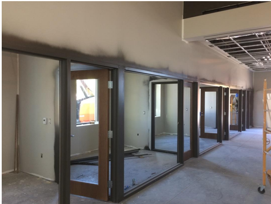
Project Site on October 23, 2018 New Study Rooms on the north side of the building.
