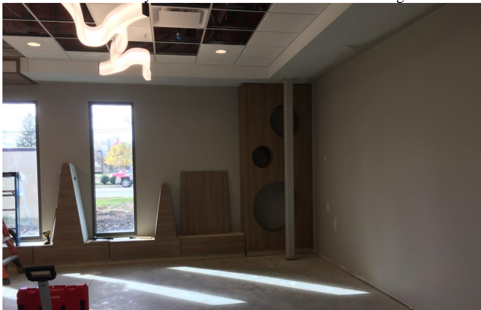
Project Site on November 6, 2018 View of the Children's Area with the window seats and light fixtures.
